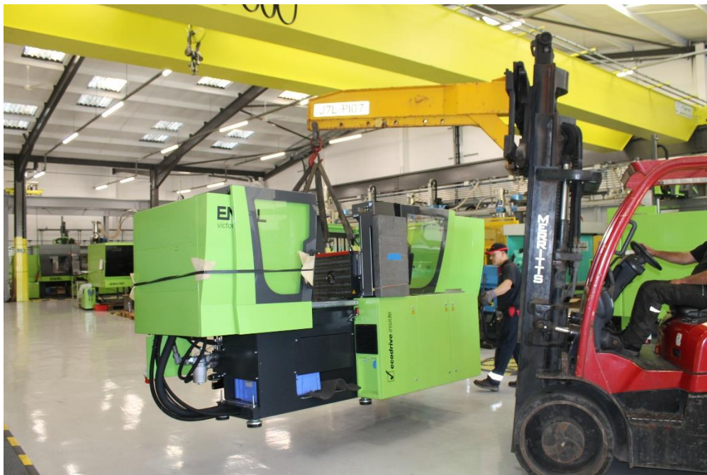
Figure 1 The new moulding machine being lifted into position at the end of 2023.
